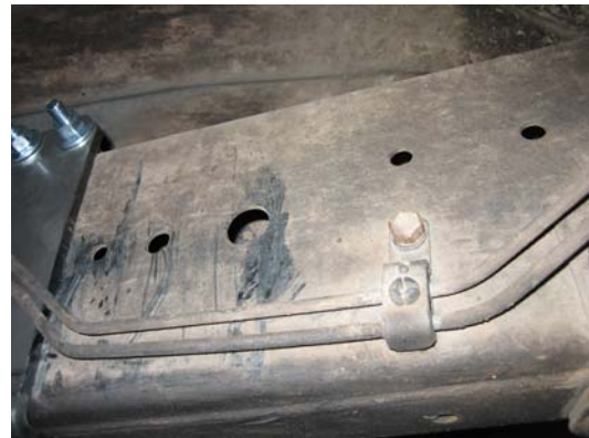
Fig 1 - Inside of Driver's frame rail
